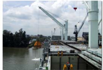
O&K Overload Test
